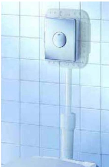
Fig. 44-A. Fluxor empotrado<sup>10</sup>.
